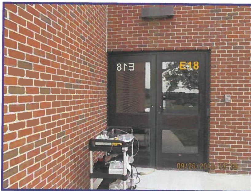
SAMPLE LOCATION ROOM # 135
